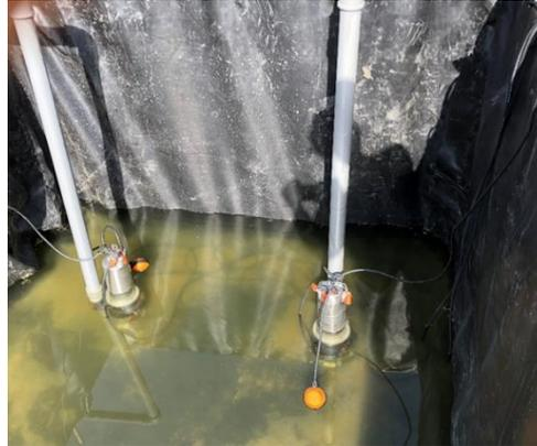
*Figura 4.* Bombas Sumergibles
